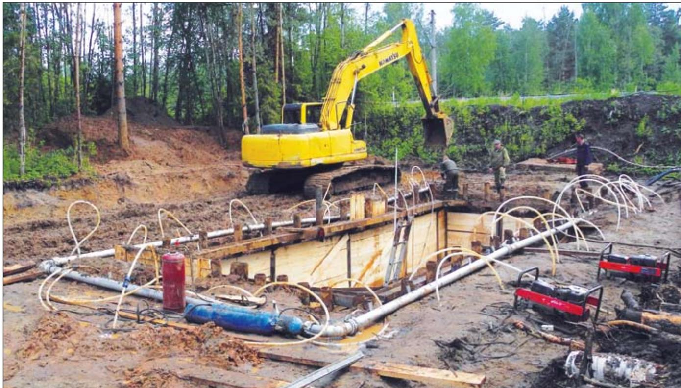
*One of the activity areas of LLC "PMK-411 "Svyazstroy" is construction of enclosed passages without trenches. The company has been working at the HDD (horizontal directional drilling) for more than 12 years. 5 complexes of horizontal directional drilling of drawbar category from 9 to 45 t allow to solve a wide range of tasks for construction of enclosed passages.*
