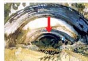
Fig. 3: Three striking cases of core-face failure followed by the collapse of the cavity in already-lined tunnels.
